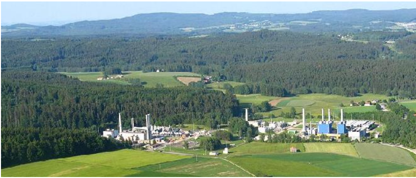
Photo 5: Compressor station in Germany containing 8 compressor units in total
