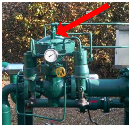
Figure 5 – Illustration of a leak to be repaired – simple case. Source: MARCOGAZ' members
