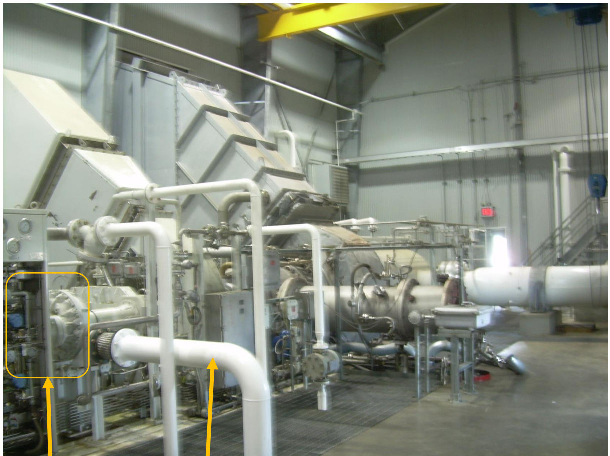
Figure 1 – Gas turbine with an expansion turbine as starting motor
