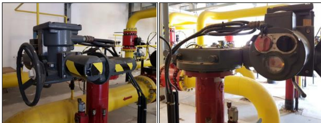
Figure 3 - Electric valves instead of gas operated valves
