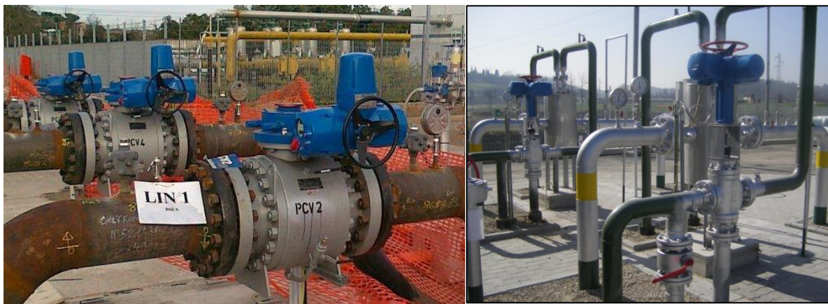
Figure 2 - Ball control valve operated by electric actuator (left) and temperature control valves with no emission (right)
