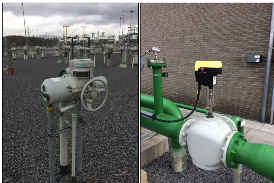
Figure 4 - Electrical actuators
