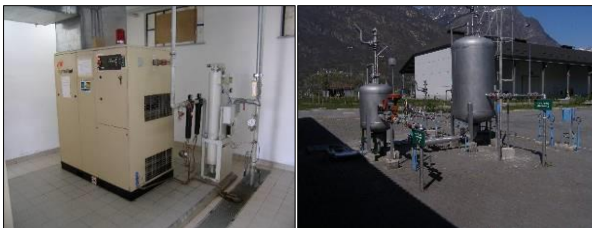
Figure 1 - Air electro-compressor (left) and air tank (right)
