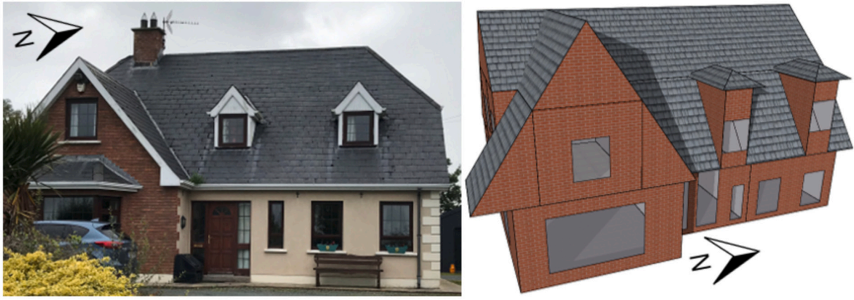
Fig. 4. Case study residential building.
